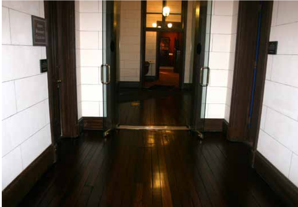
Re-finished floors in the front hall.
